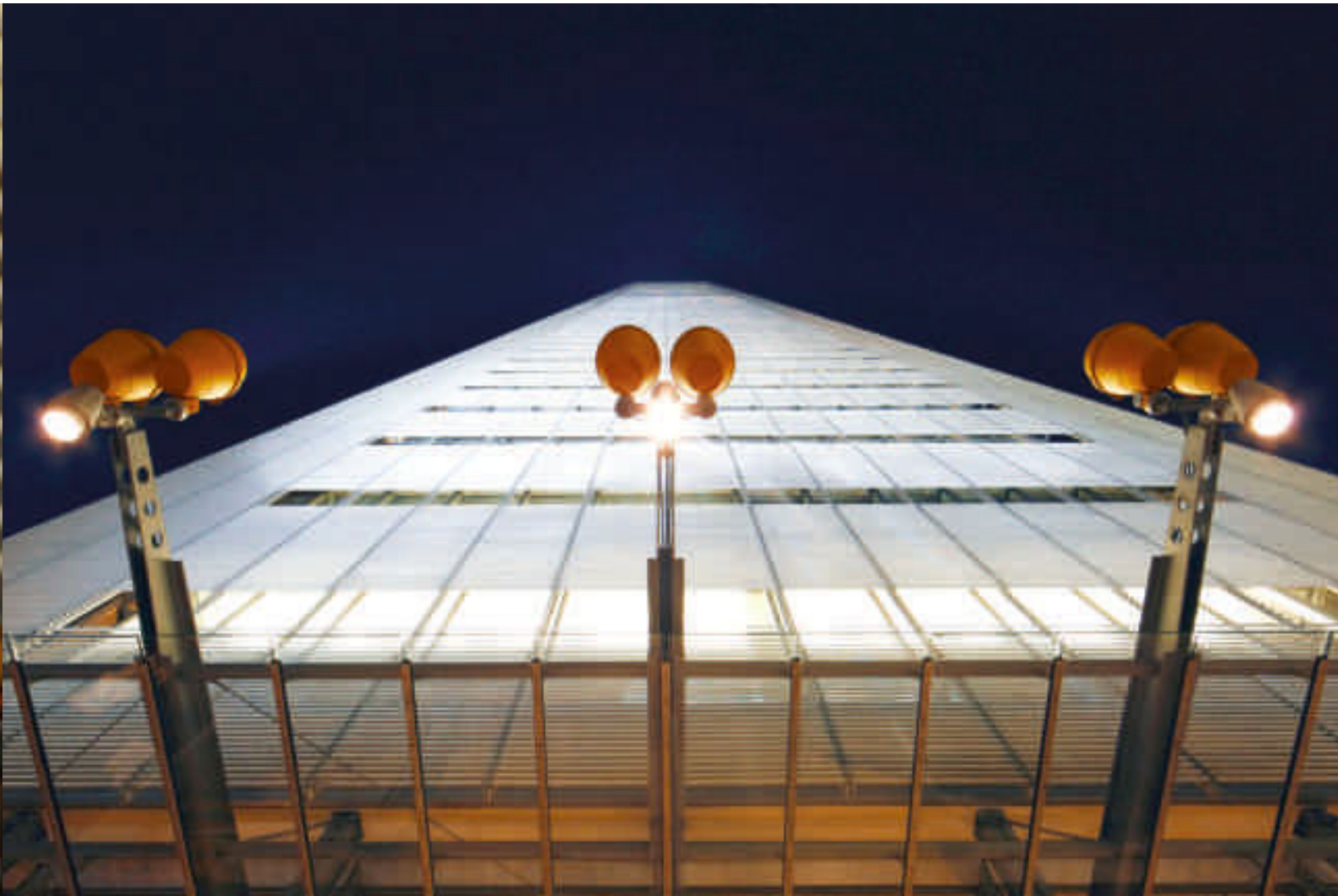
Opposite: Laser aiming of luminaires to pre-determined façade locations Above: Exterior product evaluation Below: Luminaires cast light up the 261 m (856') façade
